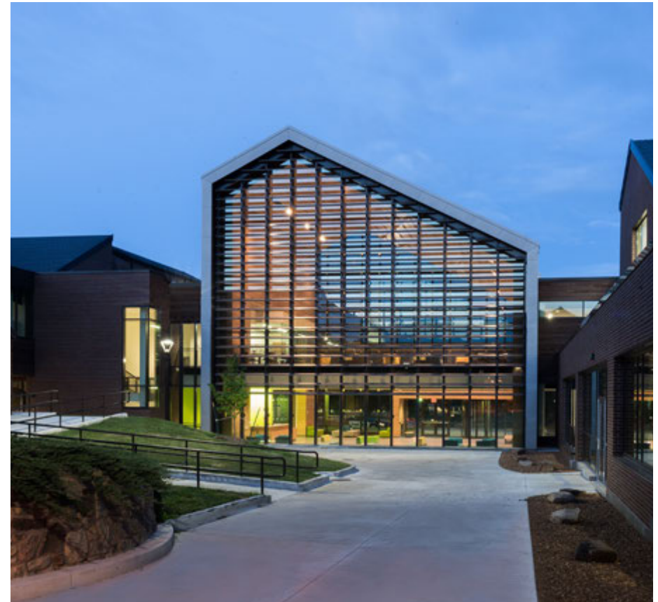
Front door atrium space (Parkland College Student Union)
